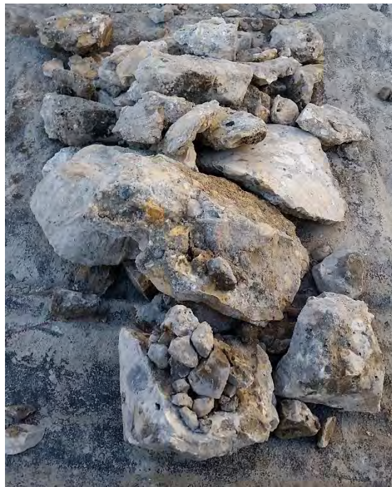
Figure 18: TH18 – 150 mm deteriorated concrete
