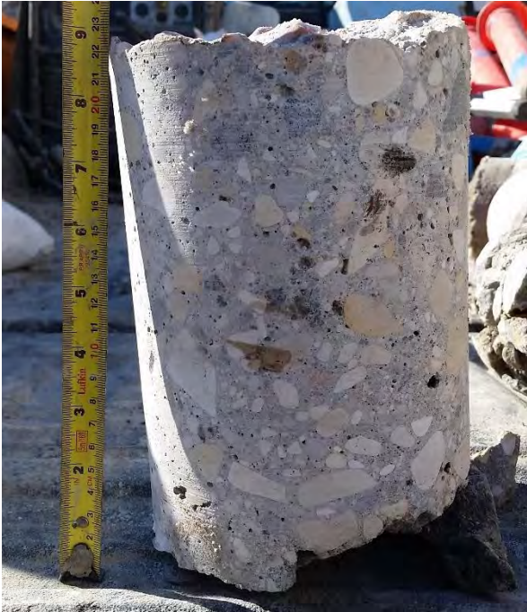
Figure 34: TH33 – 220 mm intact concrete
