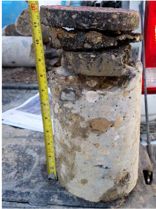
Figure 25: TH25 – 100 mm asphalt, 200 mm intact concrete
