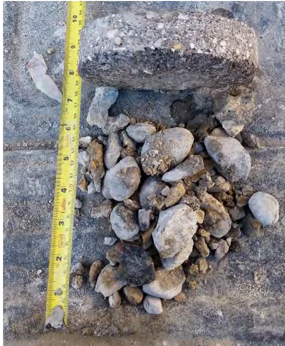
Figure 23: TH03 – 30 mm asphalt, 120 mm deteriorated concrete
