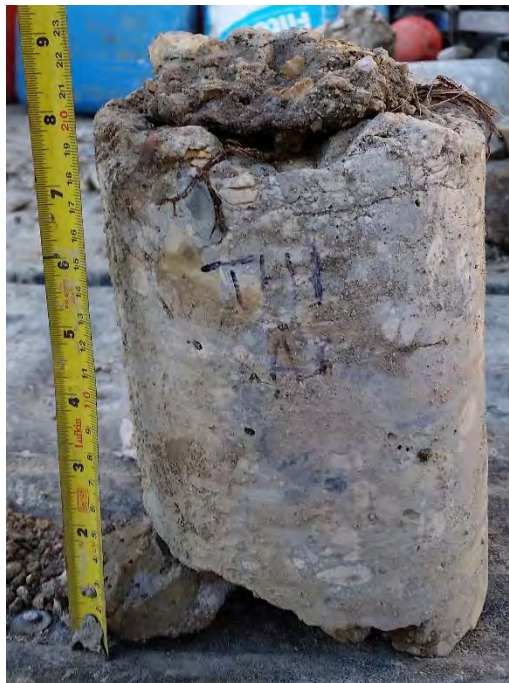
Figure 24: TH24 – 200 mm intact concrete
