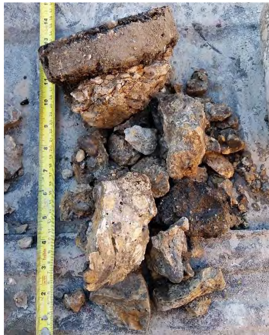
Figure 8: TH8 – 50 mm asphalt, 150 mm deteriorated concrete
