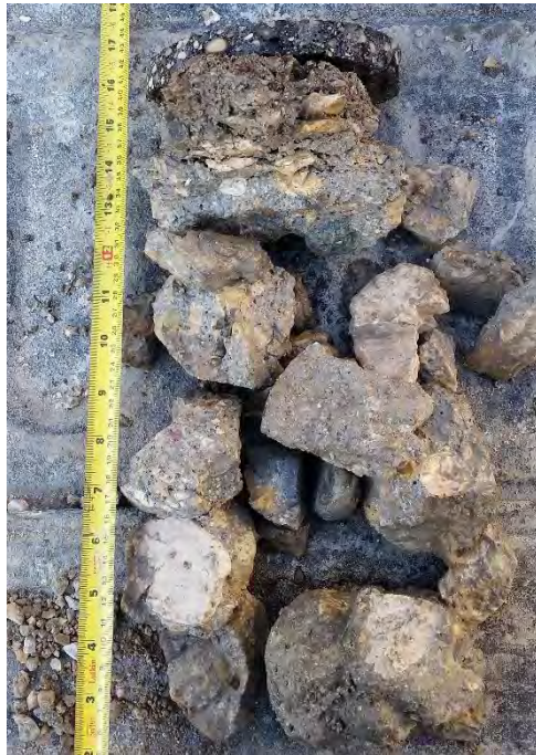
Figure 26: TH26 – 20 mm asphalt, 160 mm deteriorated concrete
