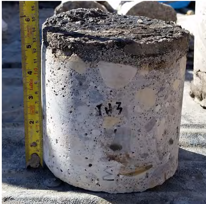
Figure 31: TH31 – 20 mm asphalt, 130 mm intact concrete
