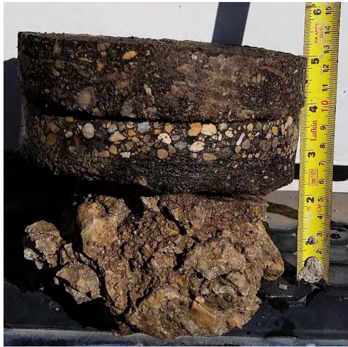
Figure 1: TH1 – 80 mm asphalt, 50 mm deteriorated concrete
