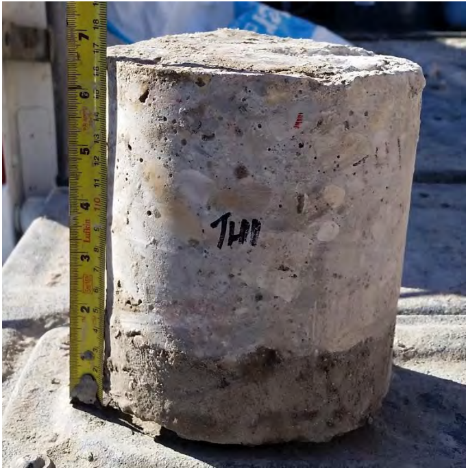
Figure 29: TH29 – 170 mm intact concrete
