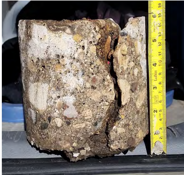
Figure 5: TH5– 150 mm cracked concrete
