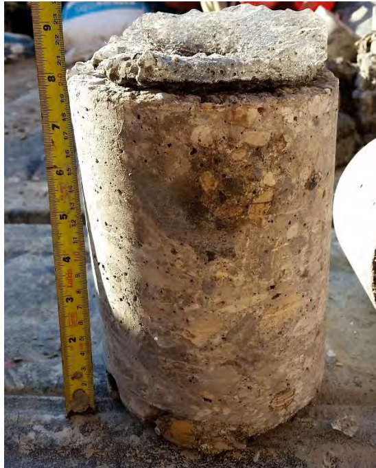
Figure 12: TH12 – 200 mm intact concrete
