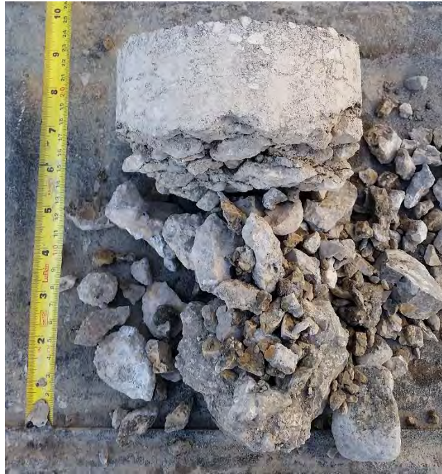
Figure 21: TH21 – 150 mm deteriorated concrete
