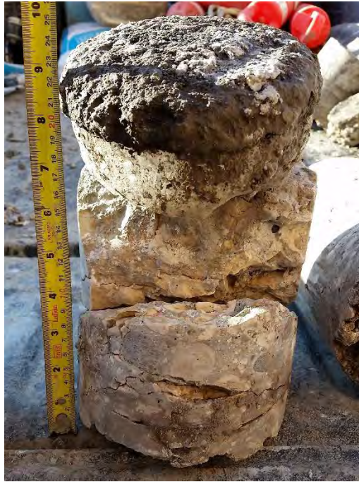
Figure 13: TH13 – 30 mm asphalt, 200 mm cracked concrete
