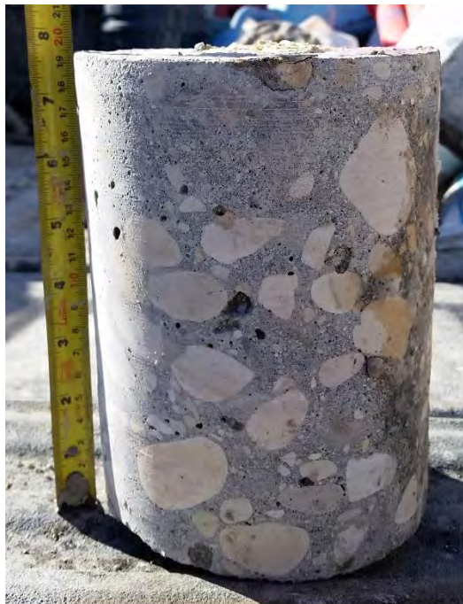
Figure 28: TH28 – 200 mm intact concrete
