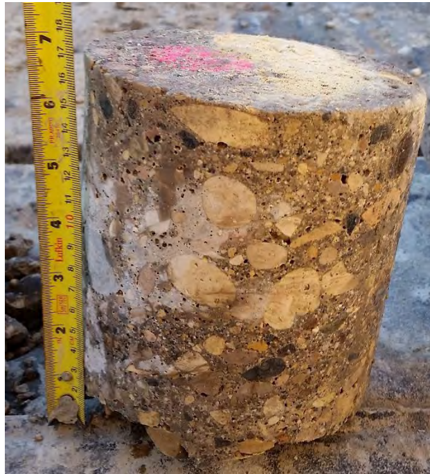
Figure 9: TH9 – 170 mm intact concrete
