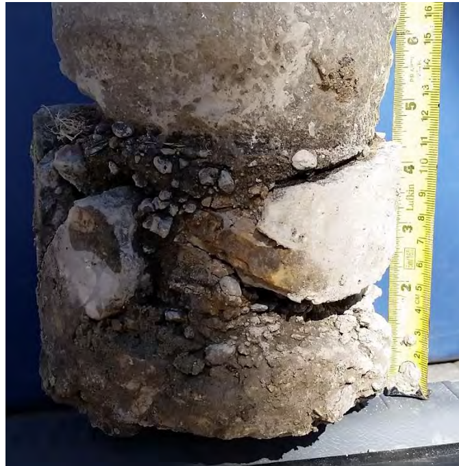
Figure 2: TH2 – 110 mm deteriorated concrete
