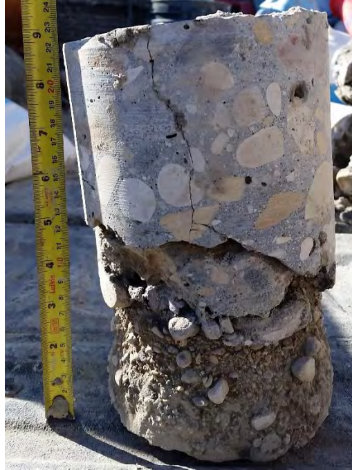
Figure 27: TH27 – 150 mm cracked concrete, 100 mm granular fill (frozen)
