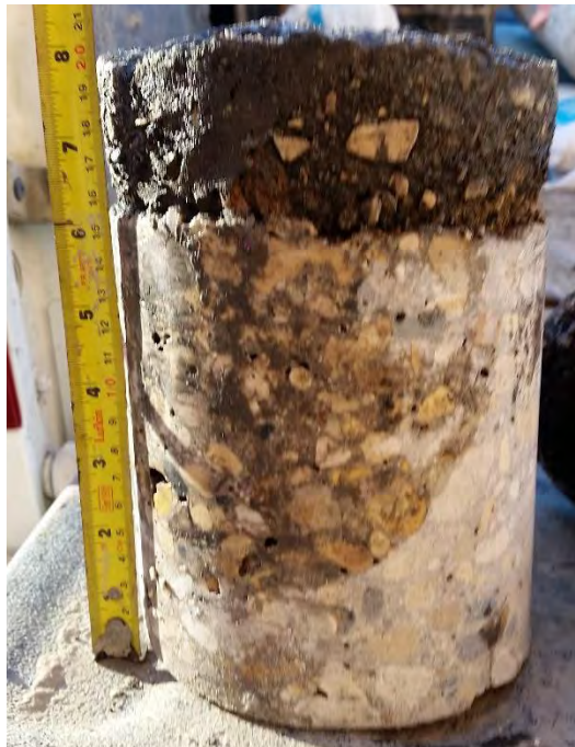
Figure 6: TH6 – 50 mm asphalt, 150 mm intact concrete
