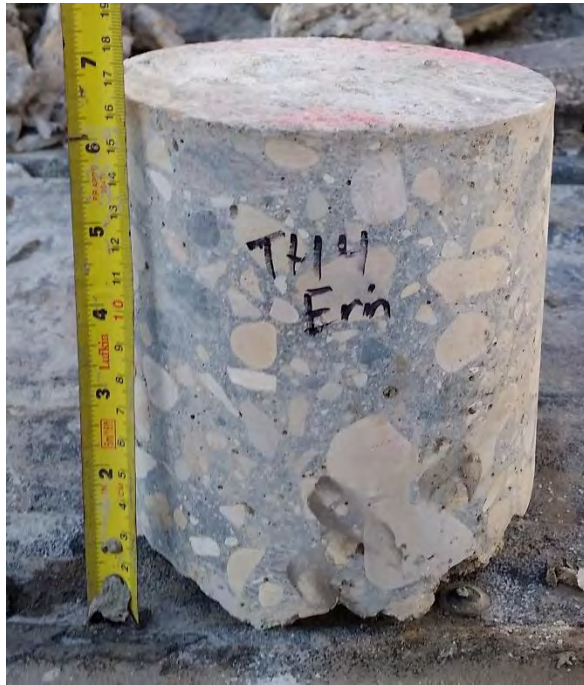
Figure 17: TH17 – 170 mm intact concrete
