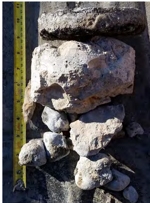
Figure 10: TH10 – 30 mm asphalt, 150 mm deteriorated concrete
