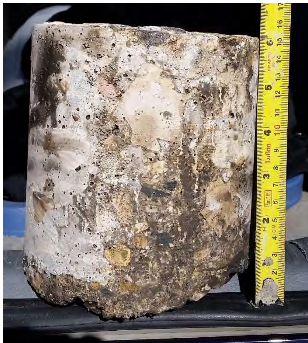
Figure 4: TH4 – 150 mm intact concrete
